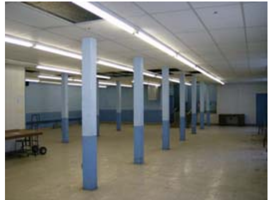
First Floor - Inside
